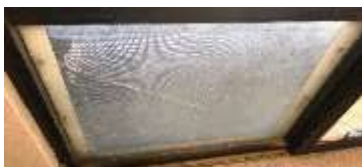
Front sliding doors.
